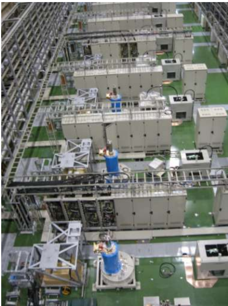
Klystron stations under construction.
