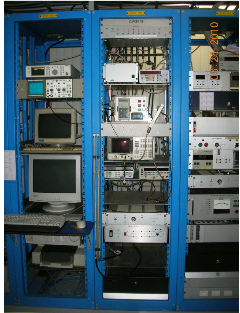
Control rack for vertical low power RF tests
