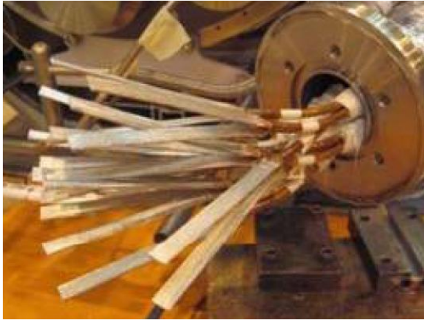
Fig. 6: Preparation of cable extremities
