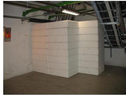
Figure 6: Shielding improvement of areas downstream the LHC injection lines [21].
