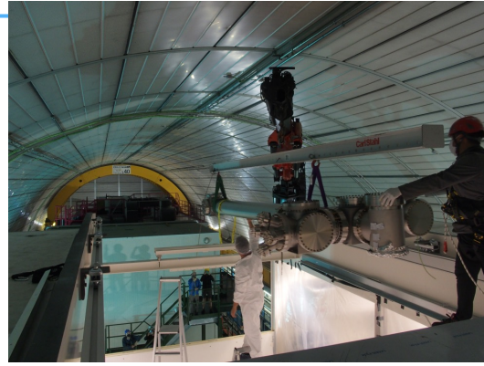
Electronics and DAQ tests Installation of mechanics and glove box
