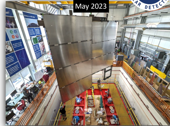
CRT north wall installation
